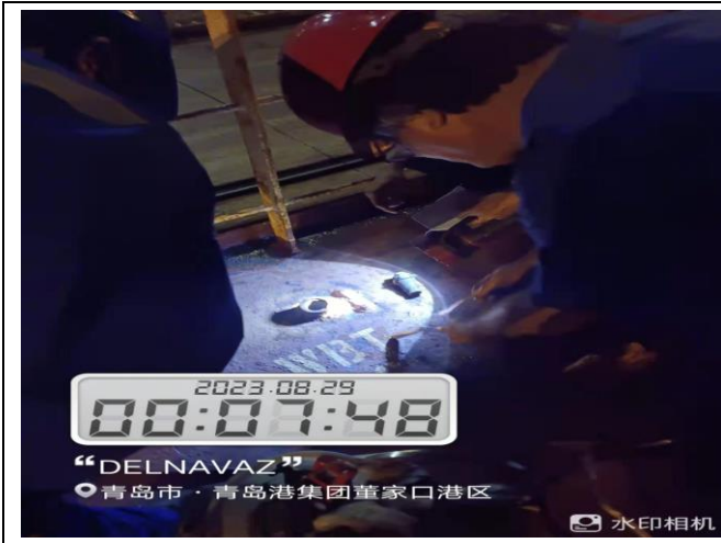
View of ballast sounding
