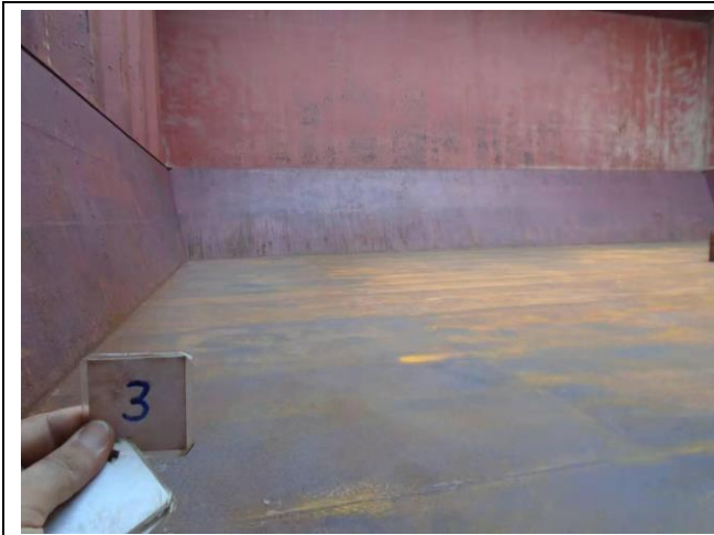
View of condition in Hold No.3
